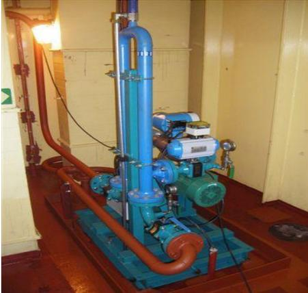
The photo above shows the additive mixing skid connected to the additive tank and the output line to the holding tank.
