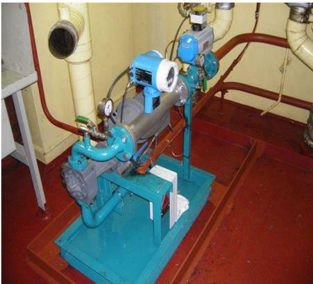
Above is the base oil pumping skid that draws in the used system oil and sends it to the additive blender. The photo below shows the input screen from the blender's control panel.
